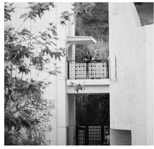
Figure 42 The new elevator tower on the left carefully matches the original facade in material, form and color, but also stands separate, minimizing its impact. 2014.
