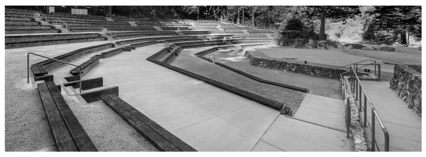
Figure 97 The original layout provided renovators with an opportunity to subtly include an "accessible" row with a wide concrete aisle and wheelchair nooks. 2021.
