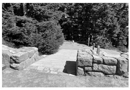
Figure 82 The 2006 renovation replaced three steps with a ramp at the amphitheater's lower entrance connecting it to a new wheelchair accessible path to the Lodge. 2021.
