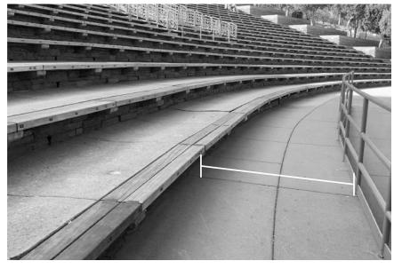
Figure 64 Renovations widened the Row 1 aisle to provide wheelchair accessible seating. 2017.
