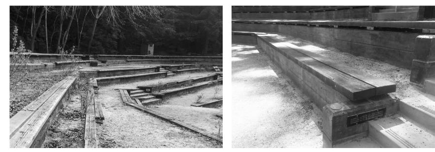
Figure 93 Just before renovation, the deteriorated benches show the impact of the wood to soil contact allowed by the original detail. 2016.
