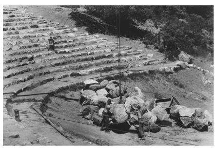
Figure 12 The Cushing Memorial Amphitheater was built by the CCC from 1935 until 1941 with most design decisions made in the field by NPS designers. Consequently, the alignment of the rows, built of on-site stones, was constantly adjusted to the topography. c. 1939.
